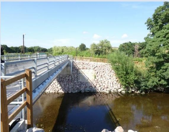
A review of the existing flood defences in St Asaph resulted in work to upgrade the defences and replace an existing bridge with a higher, wider structure.
