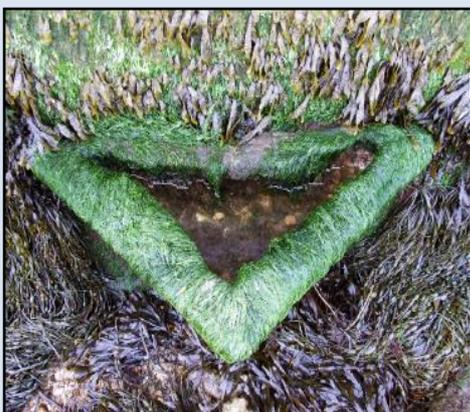
They provide an artificial rock pool which retain water as the tide recedes providing a habitat for fish and invertebrates. Marine life which colonise the pools can also strengthen the integrity of the structure and improve its resilience by providing a covering of organisms such as barnacles, mussels and seaweeds. They are also used for educational purposes allowing local school children on fieldtrips to undertake rock pooling activities and learn about marine biology.
