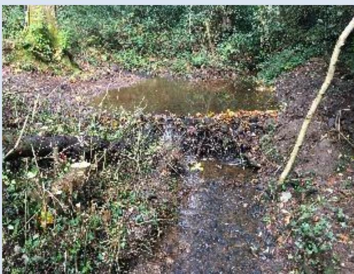
Prior to the scheme, the culvert system could not cope with flows and was blocking due to silt and stone washing downstream. The works undertaken involved the construction of leaky dams, straw bale dams and willow structures to slow down the flow of water. Block stones have also been installed to reduce the force of the water and prevent erosion of the embankments.
