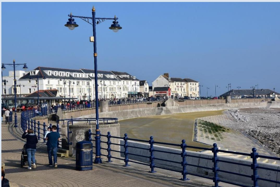
The public were consulted throughout the process and helped shape decisions on access and aesthetic elements of the scheme. The new structure is made up of 5 interlocking pre-cast concrete sections in the form of a terrace, the toe of which is protected by rock armour.
