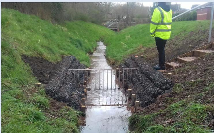
Through the Small Scale Works Grant 2018/29, Monmouthshire County Council accessed funding to deal with a surface water flooding issue around the Rockfield Estate in Monmouth. Flooding had occurred as a result of blockages to the main trash screen over a culvert.
