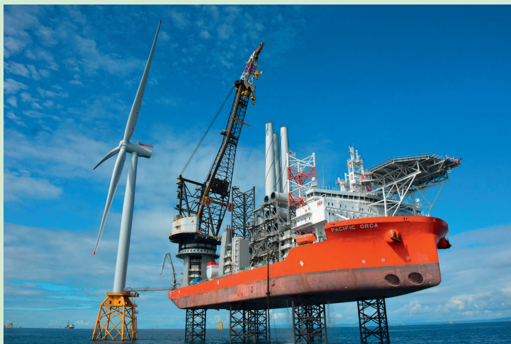
Pacific Orca installation vessel (Image: JBray)
