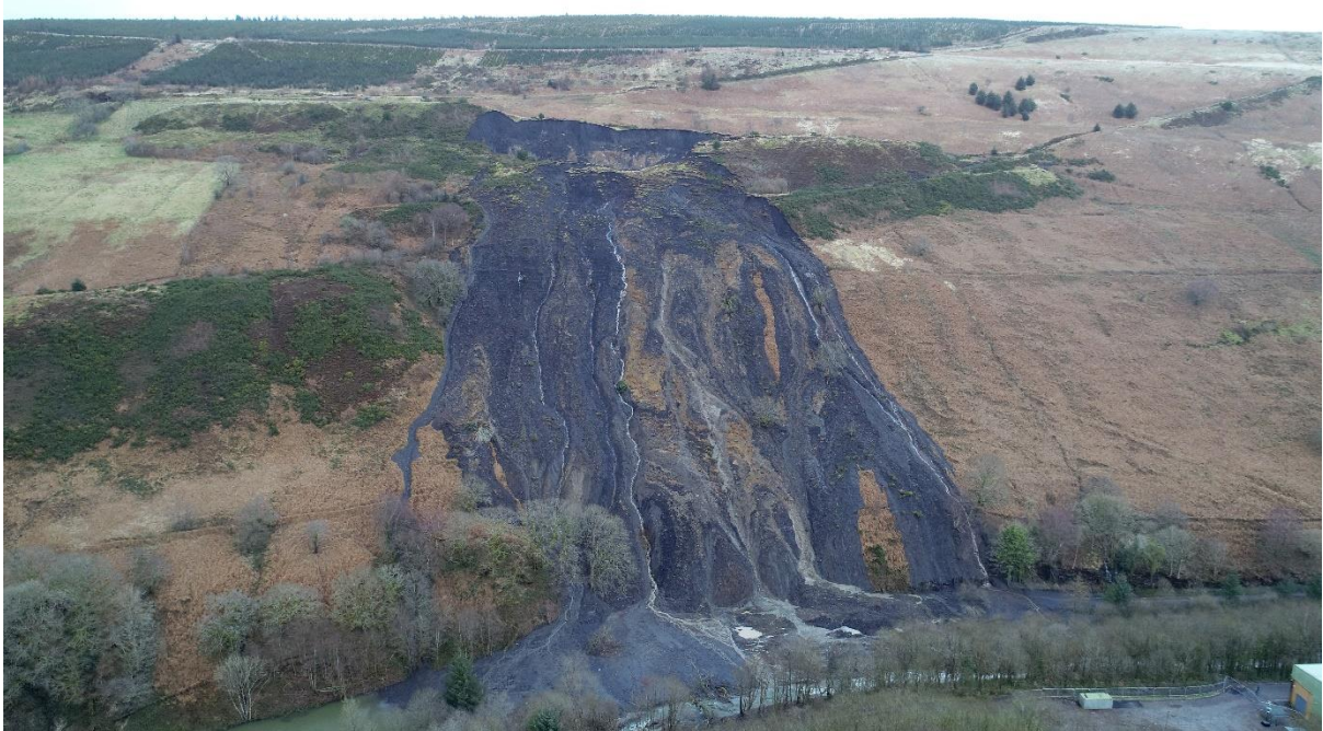
Figure 1: Thousands of tonnes of coal tip waste on the hillside and in the river at Tylorstown following the landslide in February 2020
