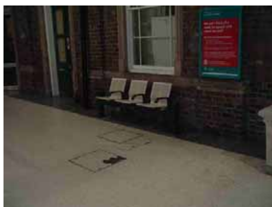
Figure 6 – Main concourse seating.
