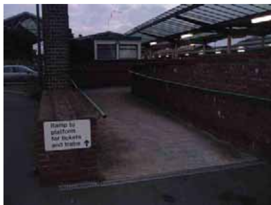
Figure 4 – Ramp from car park.
