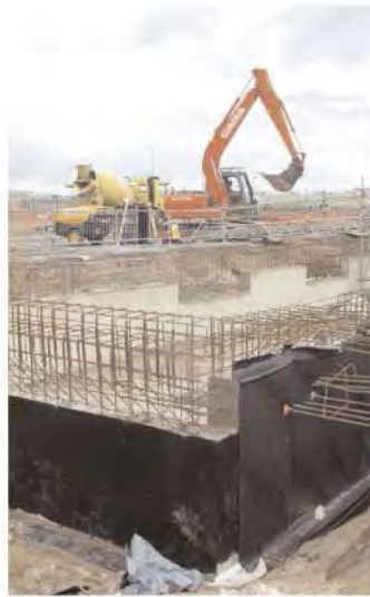
The foundations of the press.
