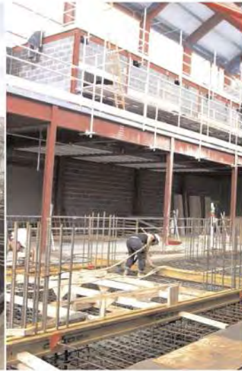
The inside of the structure starts to take shape.
