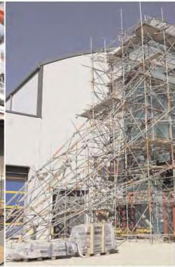
The scaffold supporting the press installation.
