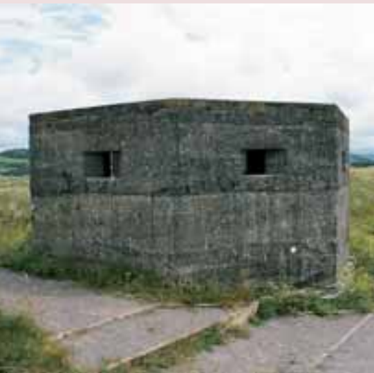
Pillbox defences at Pembrey, Carmarthenshire.
