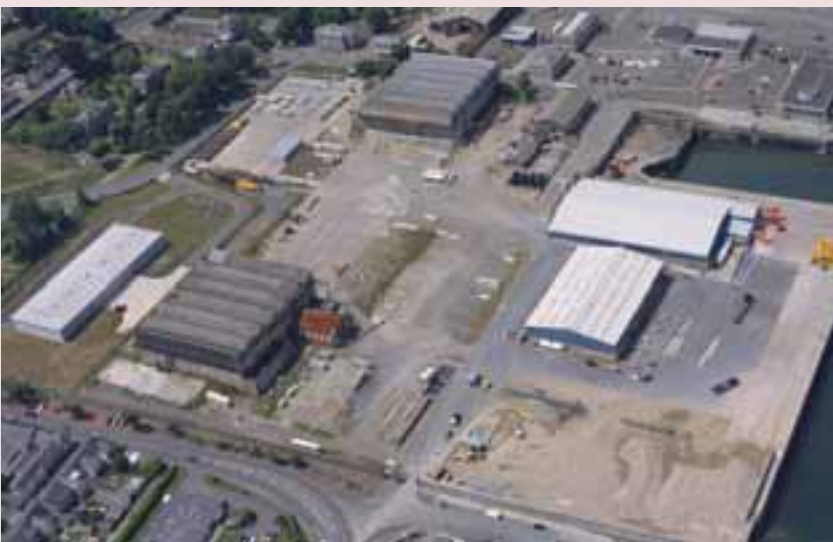
The flying boat hangars, surrounded by more recent buildings, at Pembroke Dock, Pembrokeshire (Crown Copyright: RCAHMW).
