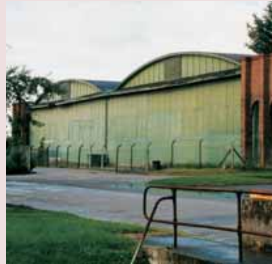
First World War hangars at Sealand, Flintshire.
