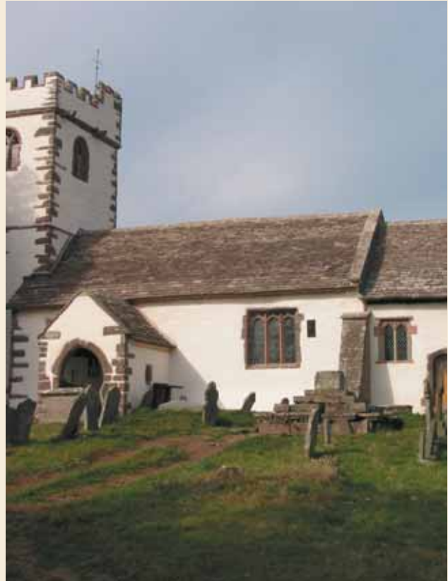
St Cadoc's Church: Decaying stonework (left) and the restored exterior (above).
