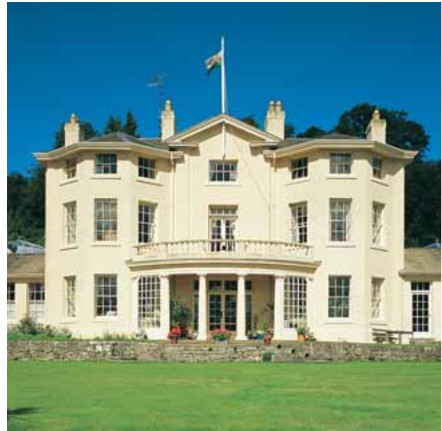
Benarth Hall, Conwy: The entrance front (opposite); the garden front before (left) and after (above) restoration.
