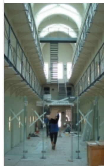
Above: The Old Gaol, Ruthin: work in progress to the interior.
