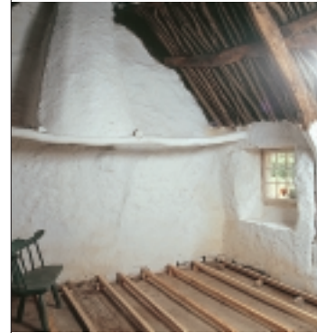
Above: The crogloft at Ffynnon Oer, Temple Bar, Ceredigion. Left: The cottage after restoration of the roof.
